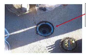
A threaded pipe plug or mechanical plug may be used to prevent water from running back into the pipe after having been drained and cleared.
