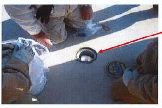
To prevent freeze expansion that could cause the can to swell and damage to concrete or the can to split, install a piece of mattress foam or Styrofoam. A 3" square is the right size for most cans.
