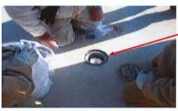
To prevent freeze expansion that could cause the can to swell and damage to concrete or the can to split, install a piece of mattress foam or Styrofoam. A 3" square is the right size for most cans.
